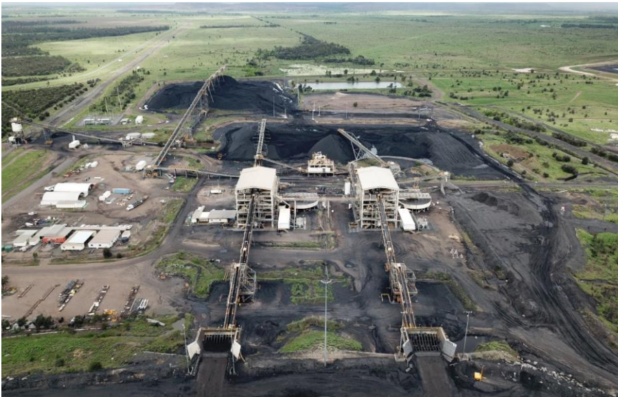
Figure 3.44: Lake Vermont Mine infrastructure
