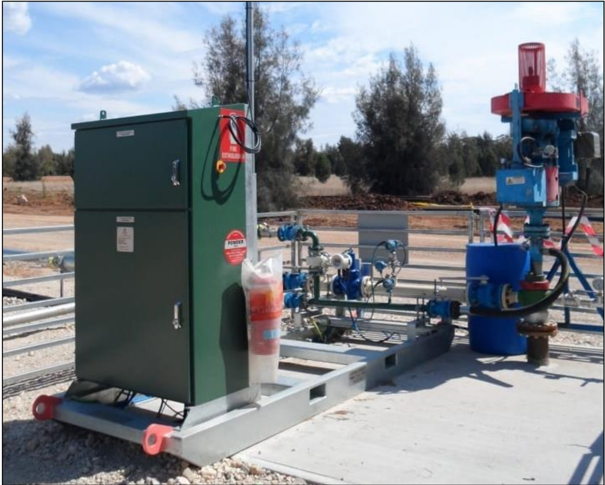
Figure 3.38: Example SIS gas drainage relocatable skid.
