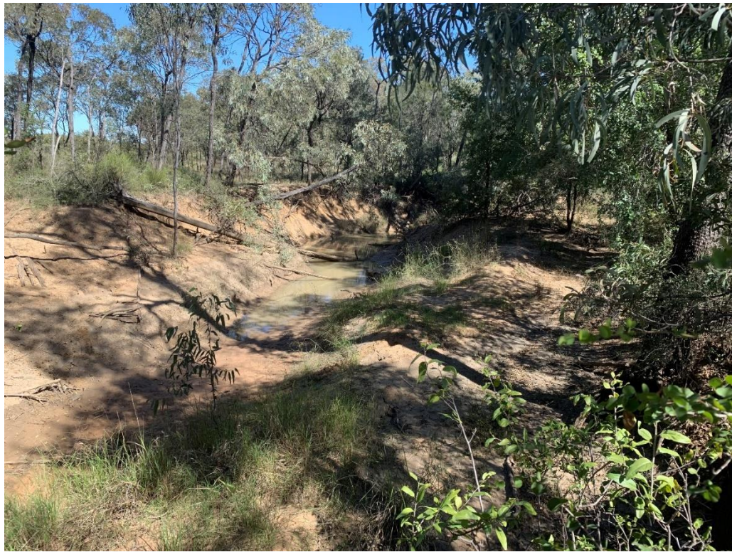
Figure 2.20 - Photograph of One Mile Creek channel (Chainage 14,075 - site O16)
