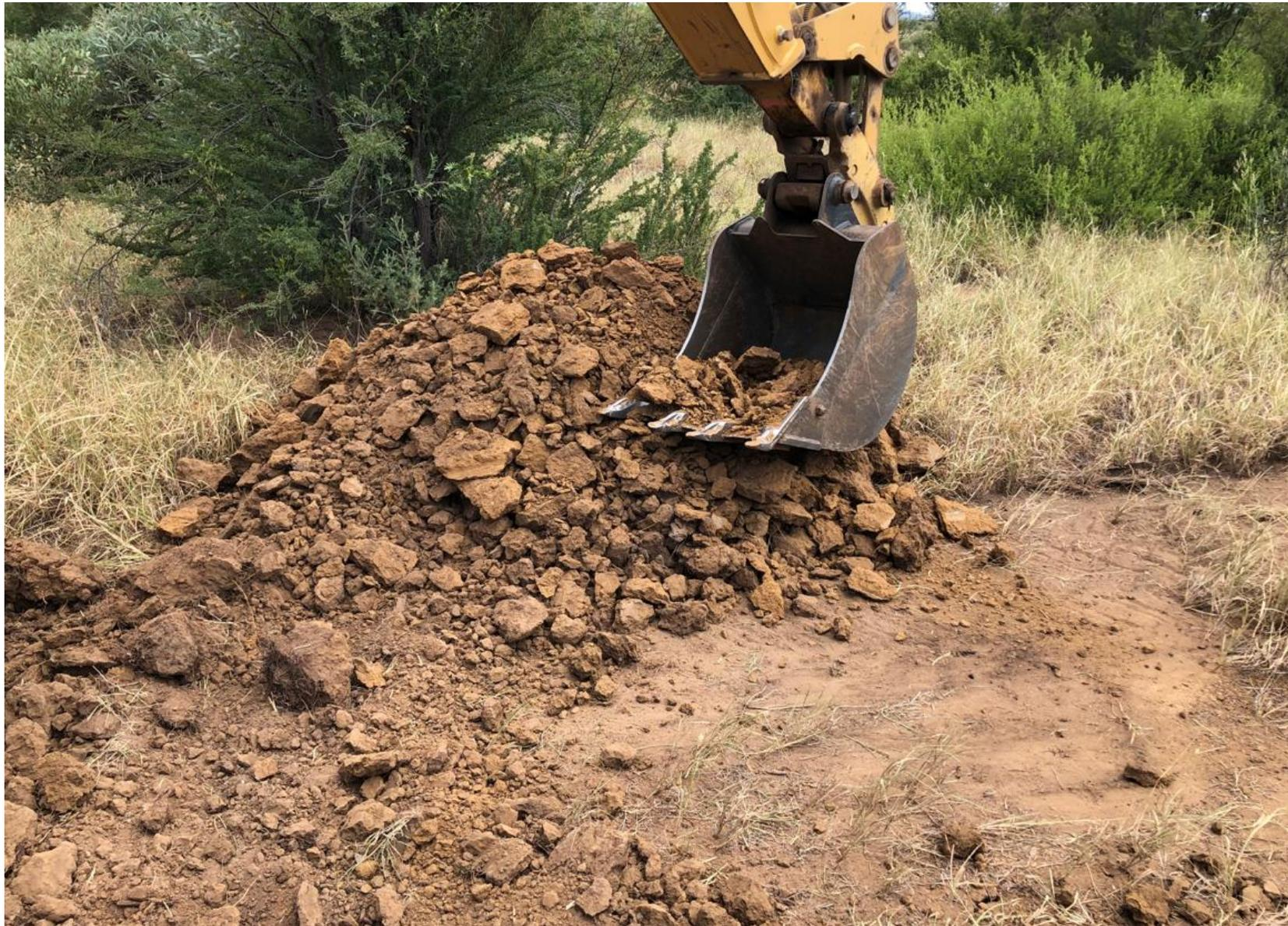
**Photo 3:** "Lumps/Clods" of clay removed from test pit
