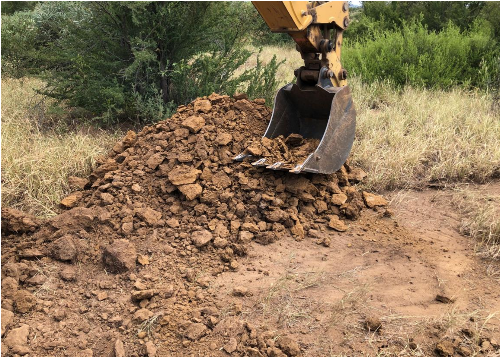
Photo 3: "Lumps/Clods" of clay removed from test pit
