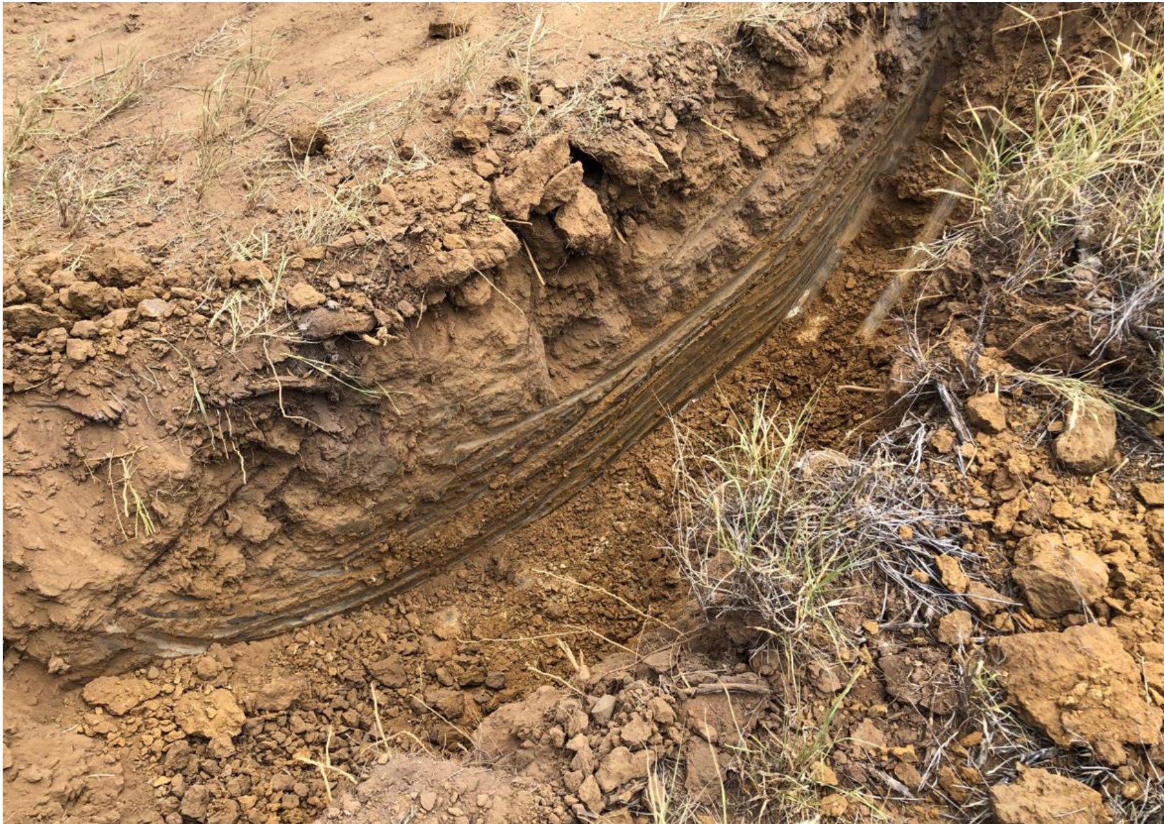
Photo 2: Typical test pit profile. Note clay “lumps/clods” and the “streaks” the excavator has imprinted into the plastic clay on sides of test pit
