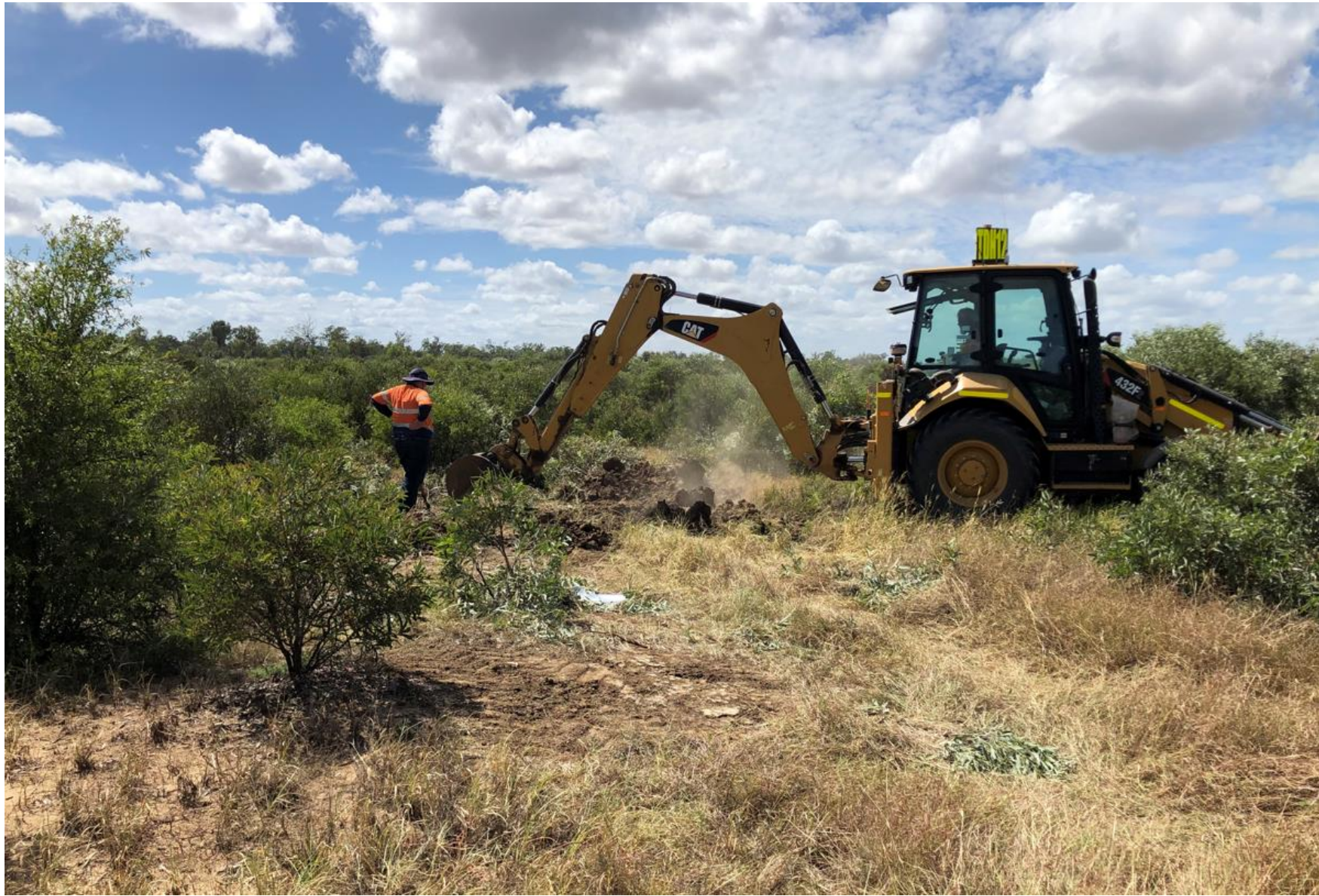
Photo 1: General Photo of Proposed Irrigation Area
