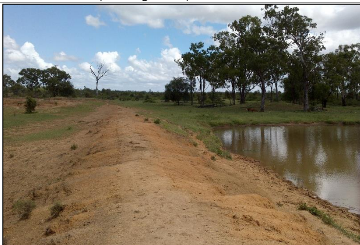
Figure 12: Typical dam within the Project area (Converge 2021).
