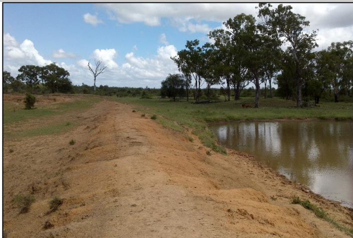
Figure 12: Typical dam within the Project area (Converge 2021).
