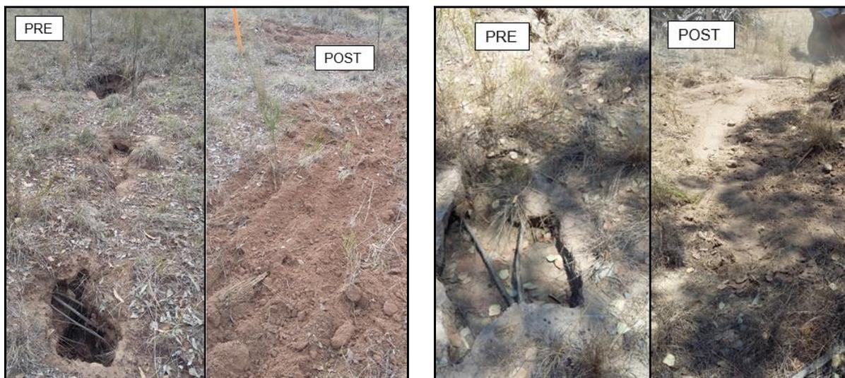
Figure 51. Examples of Crack Rehabilitation at Grasree Mine (GGPL, 2020).
